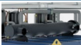
Shell and tube evaporator.
