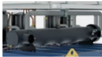
Shell and tube evaporator.
