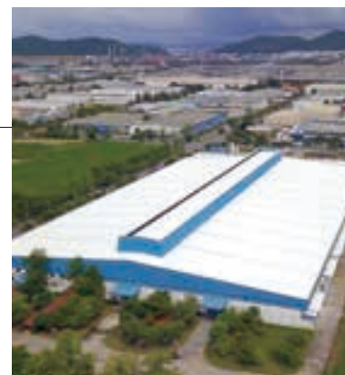
Fujitsu General (Thailand) Co., Ltd. (Thailand) Factory-2
