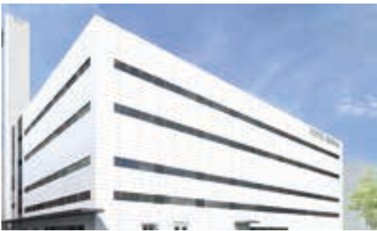
Technology research building (Japan)
