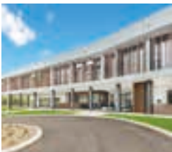
Fujitsu General (Aust.) Pty Ltd. (Australia)
